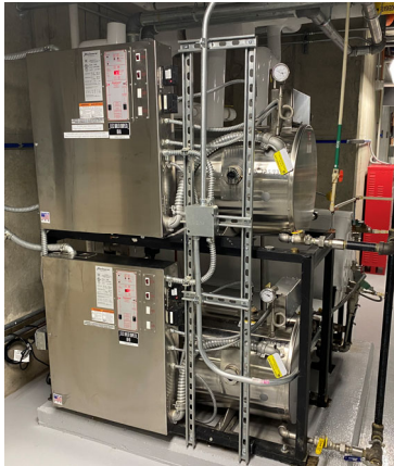
Boiler system (left and center) and steam grid (right)
