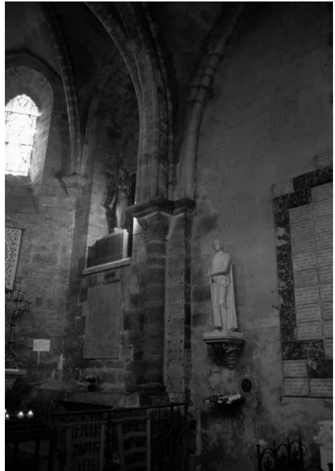
Figure 8. Notre-Dame d'Étampes, a twelfth-century dosseret and colonette of the northwest nave aisle chapel supporting a thirteenth-century transverse arch. Photo by author.
