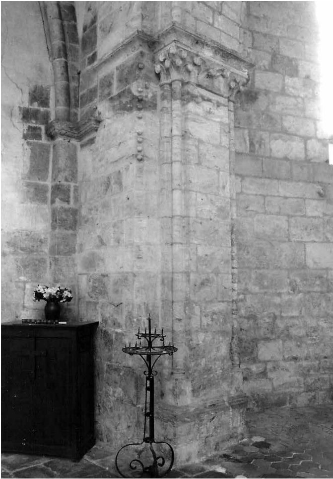
Figure 7. Notre-Dame d'Étampes, interior of the southwest nave chapel, south side, showing an embedded dosseret and impost with thirteenth-century masonry additions, including crocket capitals and ball moldings. Photo by author.
