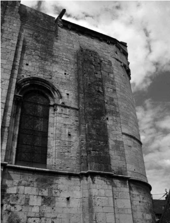
Figure 11. Southeast end of Notre-Dame d'Étampes, showing the wall extension above the south choir aisles; the ball molding is at the upper center. Photo by author.
