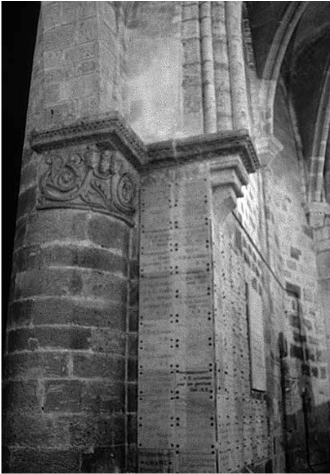
Figure 9. Notre-Dame d'Étampes, north nave aisle chapel, south side: the twelfth-century nave pier with an impost extension to receive the thirteenth-century transverse arch; break visible to the right of the large capital. Photo by author.
