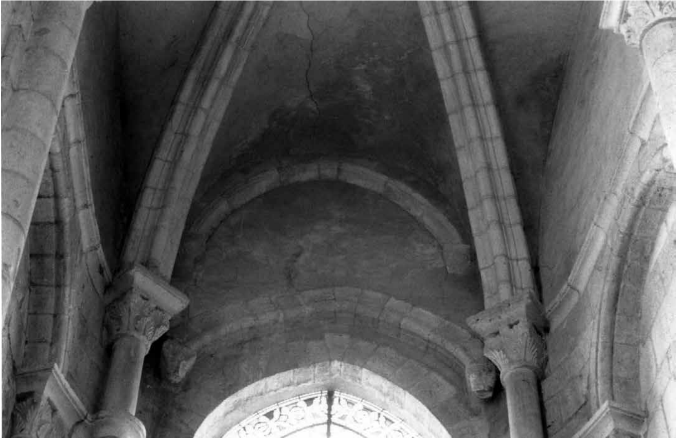
Figure 15. Notre-Dame d'Étampes, capitals and rib vaults of the northeast choir aisle chapel. Photo by author.
