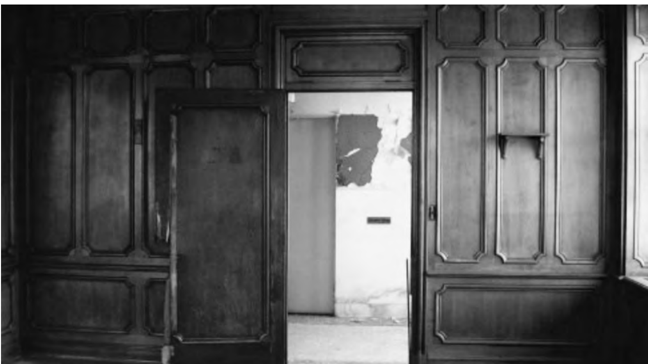
Wood paneling will be re-purposed and used for the security desk in the lobby in order to preserve the history of the building by using the original material.
